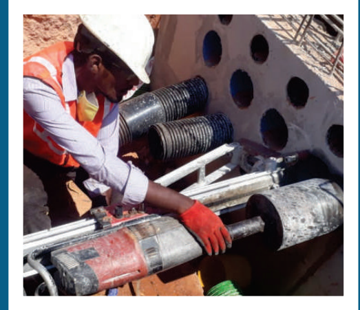
RCC Core Drilling
