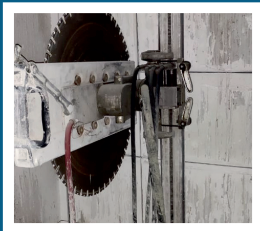
RCC Diamond Cutting
